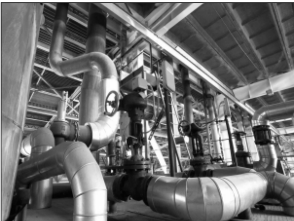
Cold Storage, Meat Processing, and Dairy
